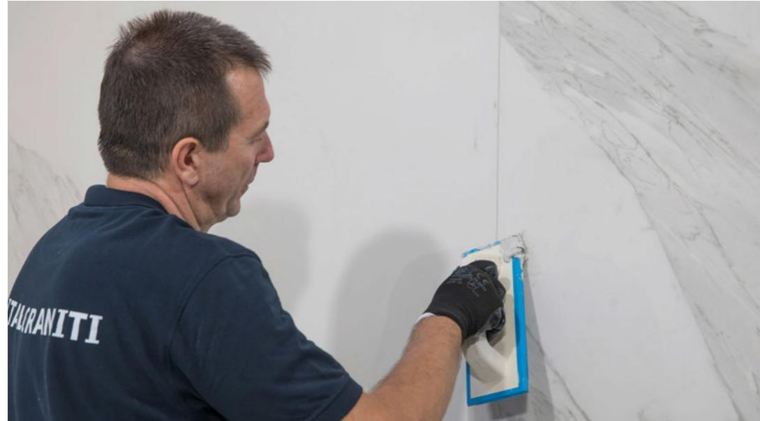
**8.** Alternate and lay out the pieces to create a natural distribution of the pattern and grains. We suggest to match grout colour with slab, using a minimum space of 2 mm when laying a single size (as foreseen by European regulation).
