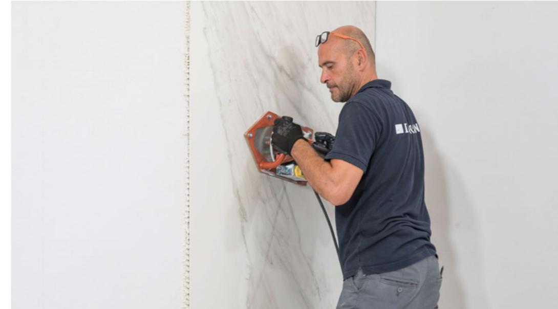
6. Use a vibrator for tiles (or alternatively a cushioned plastic hammer) to make sure that the slab is glued evenly to the substrate. Tap from the centre to the edges to assist the venting of any air pockets between the slab, the adhesive and the substrate. Do not use hammers or unsuitable tools.
