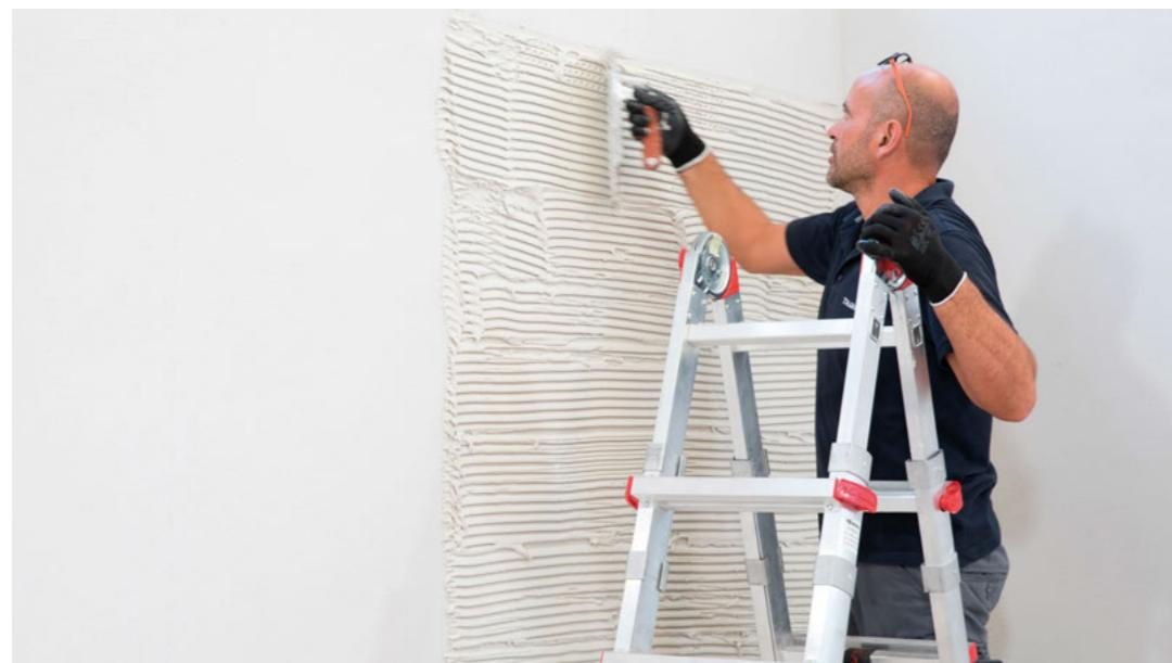
**2.** Apply the glue to the wall using a serrated trowel with slanted teeth (10x10 mm), spreading the adhesive 5/10 cm beyond the edges of the slab.
