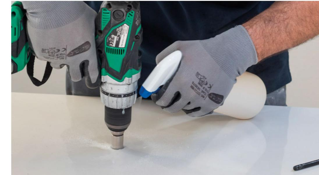
**3.** Keep the drill/screwdriver at an angle of 90° and, applying gentle, constant pressure, make circular movements at an angle of about 5°-10°.
