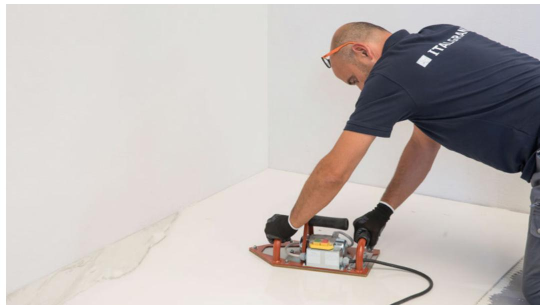
6. Use a vibrator for tiles (or alternatively a cushioned plastic hammer) to make sure that the slab is glued evenly to the substrate. Tap from the centre to the edges to assist the venting of any air pockets between the slab, the adhesive and the substrate. Do not use hammers or unsuitable tools.
