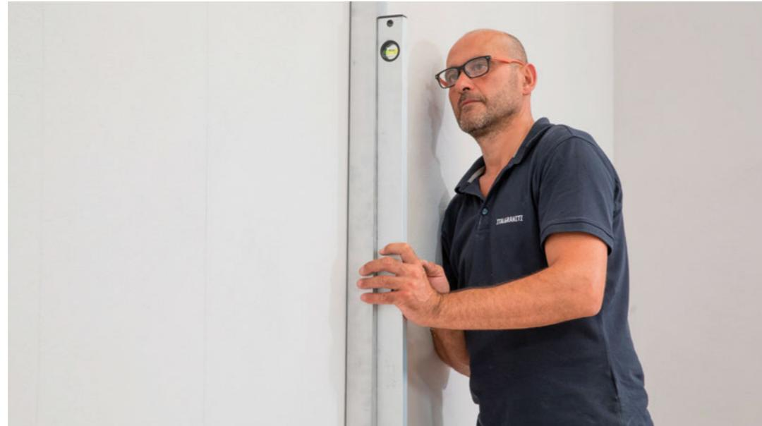
**1.** Before proceeding with final installation, check that the substrate is perfectly flat, dry and clean. Use the adhesives described, mixed in accordance with the instructions provided in the relevant technical information. High performance cement adhesives in class C2 or above should be used. An adhesive with no vertical slip (this characteristic is identified by the letter T) should be used.
