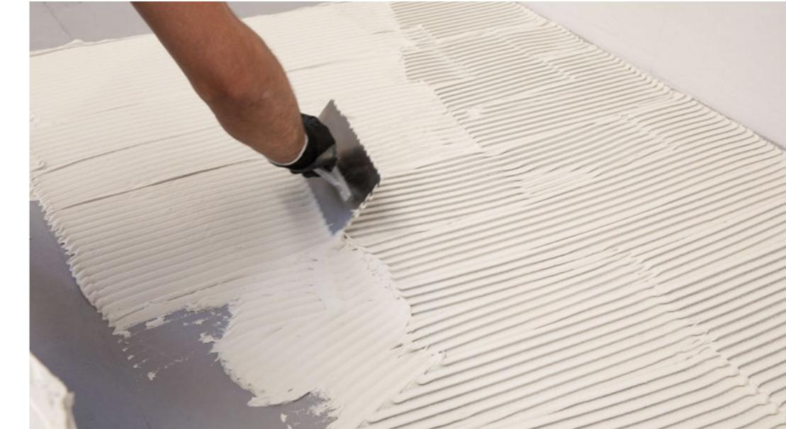
**3.** After applying the adhesive, make sure that all the lines created by the last pass of the trowel run in the same direction (theoretically, the lines should be parallel to the short side of the slab), taking care to avoid criss-cross lines, which tend to trap air in the centre of the slab.
